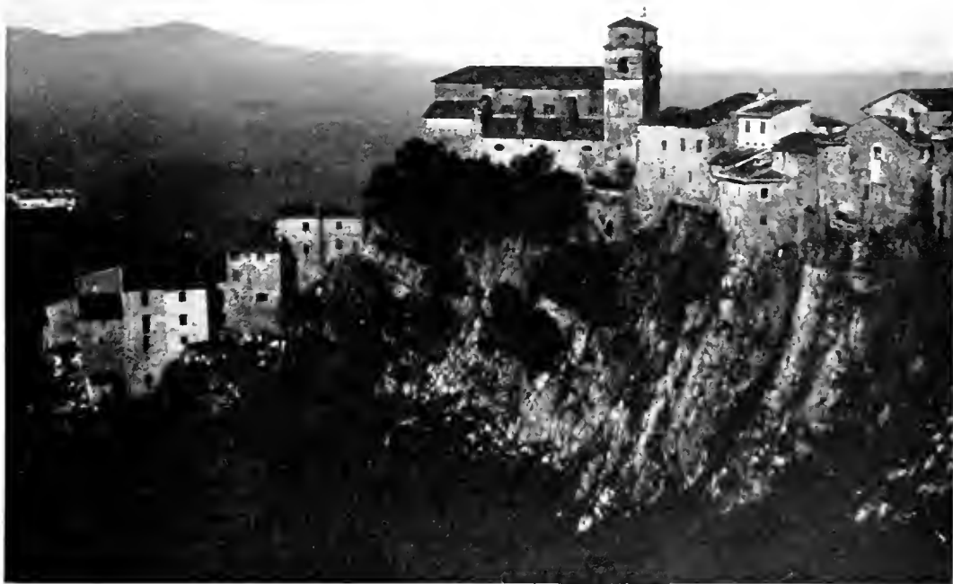
FIGURE 16. — VIEW OF ARTENA FROM THE ROAD LEADING TO LA CIVITA It shows the deep fissure west of the church, and the Albau Hills in the distance
